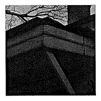
Fascia board is rotten on the roof stoop coming off the back door of the main house. This door lines up with the exterior cook house and the deterioration is on the front right side of the stoop.
