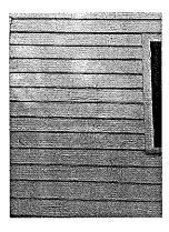
On the church side of the house, there are about 3 boards that the paint is bubbling up on. The specific area is situated above, below and between the dining room window and kitchen windows.
