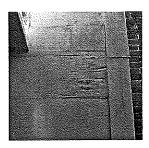
On the front right side of the house, there is a rotten spot where the side skirting of the porch roof attaches to the body of the house.
